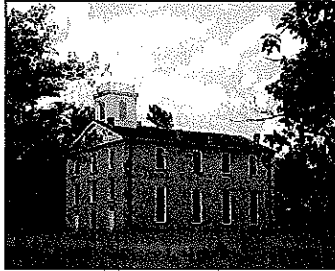
Eleutherian College Classroom and Chapel Building National Park Service
