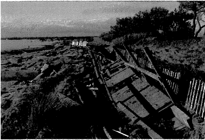
Figure 17.17 Storm damage on a coastal dune. This boardwalk, on a beach on the Atlantic Coast of France, demonstrates the force of a coastal storm. Without sand dunes, the force of storms is directed inland, often in developed areas.
