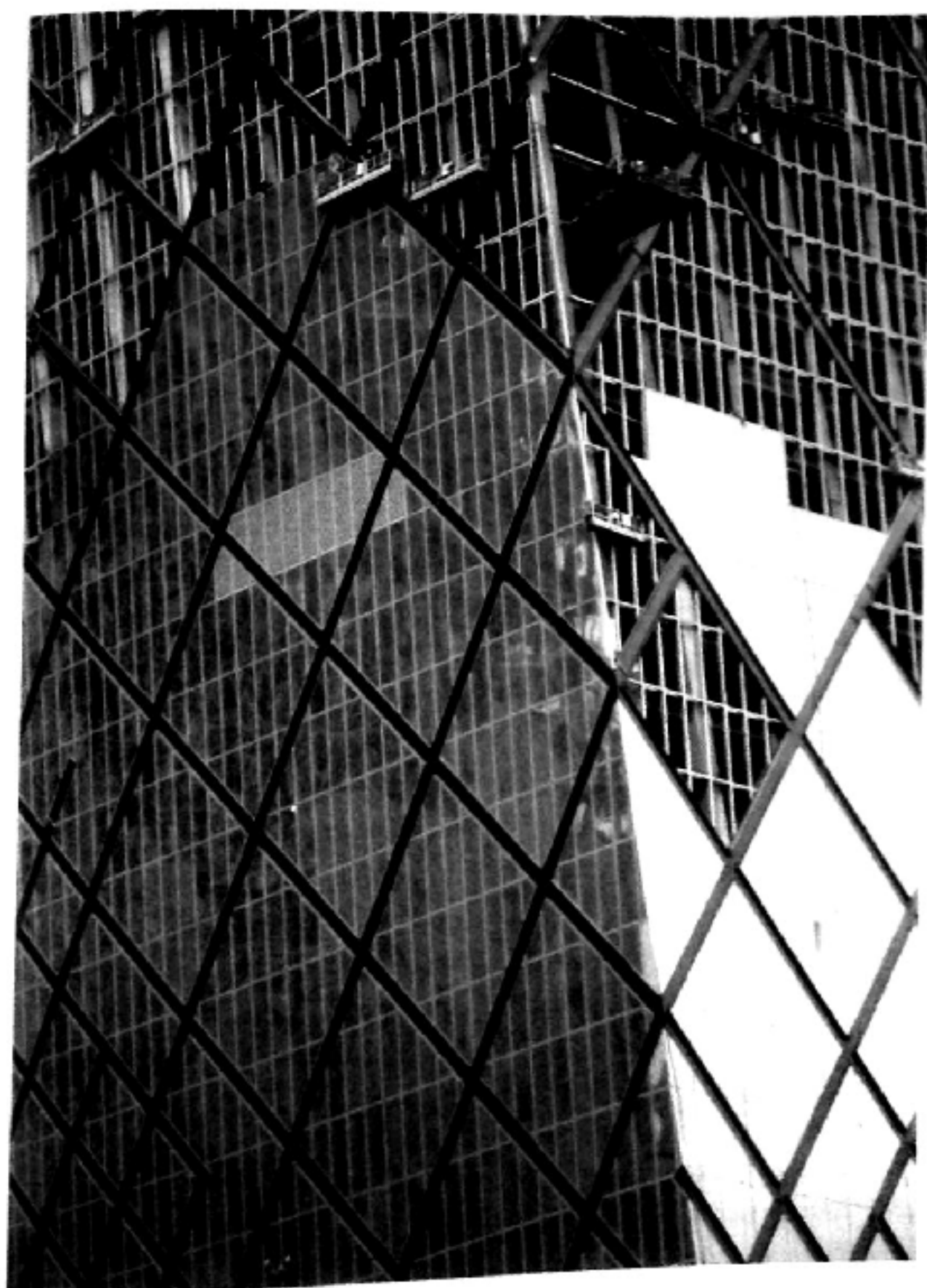
Figure 12 OMA/Rem Koolhaas, construction detail, CCTV Headquarters, Beijing, 2002–12, photo: Ana Abram, 2008.
