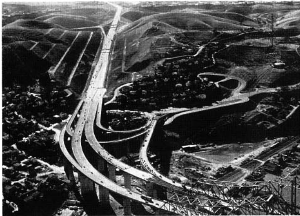
BELOW: Carquinez Bridge Approach, Crockett, California, 1958
