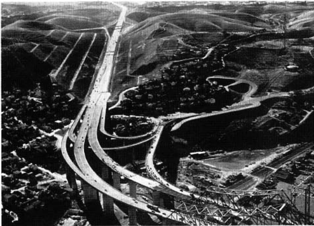
BELOW: Carquinez Bridge Approach, Crockett, California, 1958
