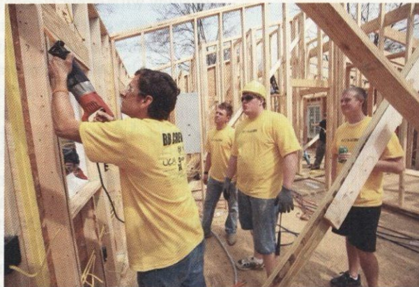
Volunteer Duane Dixon, on the left, cuts through a stud while other volunteers look on. These individuals volunteered to help build and furnish a home in five days for a wheelchair-bound woman in Alabama.
