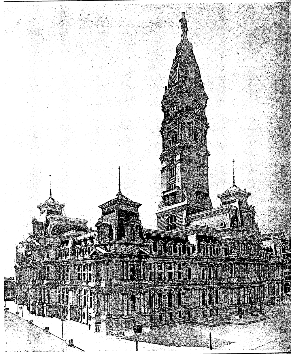
Philadelphia City Hall, Centre (Penn) Square, site preparation and construction 1870-1901, designed by John McArthur, Jr. (1823-1890), photograph 1899. The view, looking toward the southwest, includes corners of the United States Mint at the left and the Pennsylvania Railroad Station at the right.
