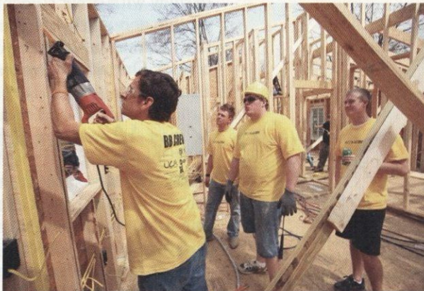
Volunteer Duane Dixon, on the left, cuts through a stud while other volunteers look on. These individuals volunteered to help build and furnish a home in five days for a wheelchair-bound woman in Alabama.
