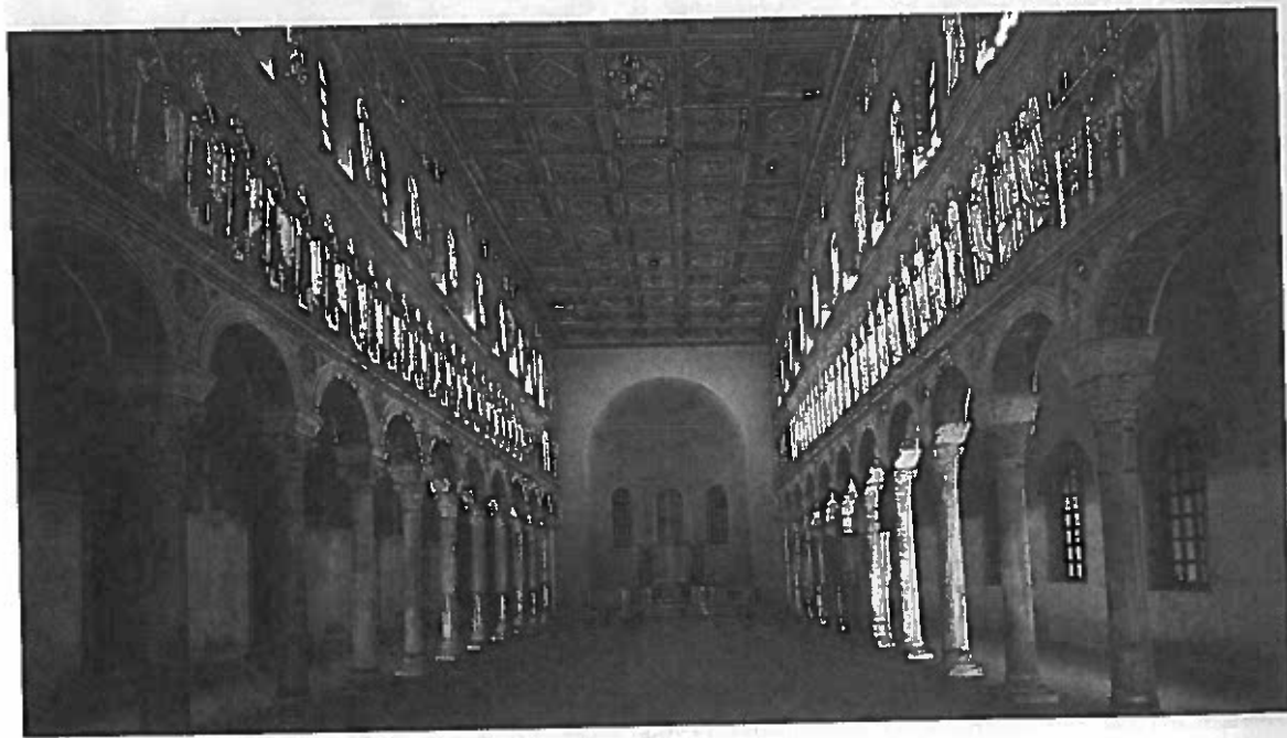
Fig. 8.24 Nave of Sant'Apollinare Nuovo, looking east, Ravenna, ca. 500 and later. The rising water table in Ravenna has caused the floor of the church to be raised four feet since the sixth century. In the process, a fourth tier of mosaics has been lost, cut out of the wall to accommodate the higher floor. It is not clear what was represented in this tier of mosaic, nor do we know what originally decorated the apse, which was also destroyed.
