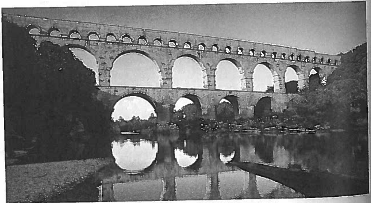
Pont du Gard, near Nîmes, France, late first century BCE–early first century CE. Height 180'. The Roman city of Nîmes received 8,000 to 12,000 gallons of water a day from this aqueduct.
