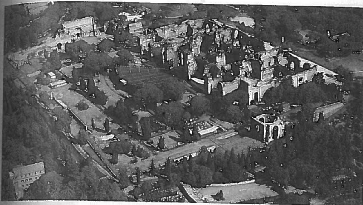
Fig. 6.30 Baths of Caracalla, Rome. 211–217 CE. Rome's baths and public waterworks required enormous amounts of water. The city's 14 aqueducts brought 220 million gallons of pure spring water per day from the Apennines, the mountain chain that extends the length of the Italian peninsula. This water supplied 11 public baths, 856 private smaller baths, and 1,352 fountains and cisterns.
