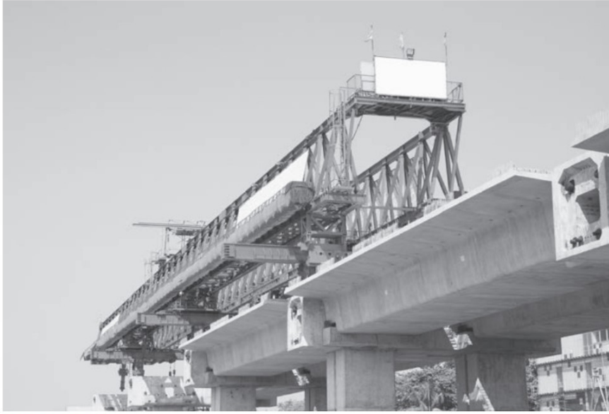
FIGURE 13.18 Honolulu's Elevated Rail project
