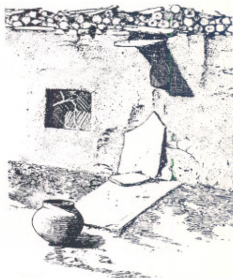
Splash blocks under Canale, Zuni
