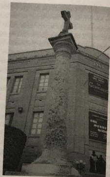
FIGURE 6.6 Erosion of carbonate column in Maltese square. (Courtesy of DHD Multimedia Gallery, http://aj.hd.org .)
