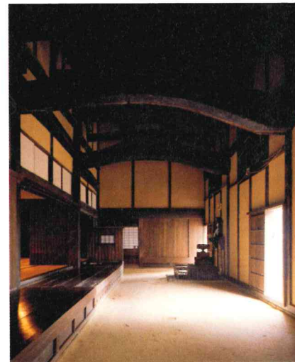
41 Traditional do-ma : the ground itself used as an enclosing element of habitable space. Kumaya House, Yamaguchi
