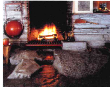
2 Integration of an existing boulder as a hearth. Frank Lloyd Wright: Fallingwater, Bear Run, PA, 1936
