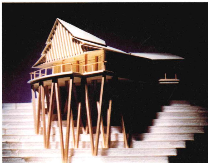
38 An updated version of the traditional kake-zukuri structure. Hidetoshi Kawaguchi's proposed new worship hall for the Temple of Shichifukuten-ji, Chiba
