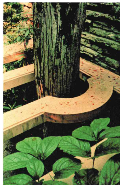
3 Accommodation of an existing tree. Frank Lloyd Wright: Fallingwater, Bear Run, PA, 1936
