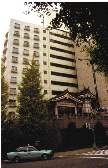
37 The ancient spirit of a place re-housed. A rebuilt Shinto shrine incorporated into a modern building, Sengaku-ji, Tokyo
