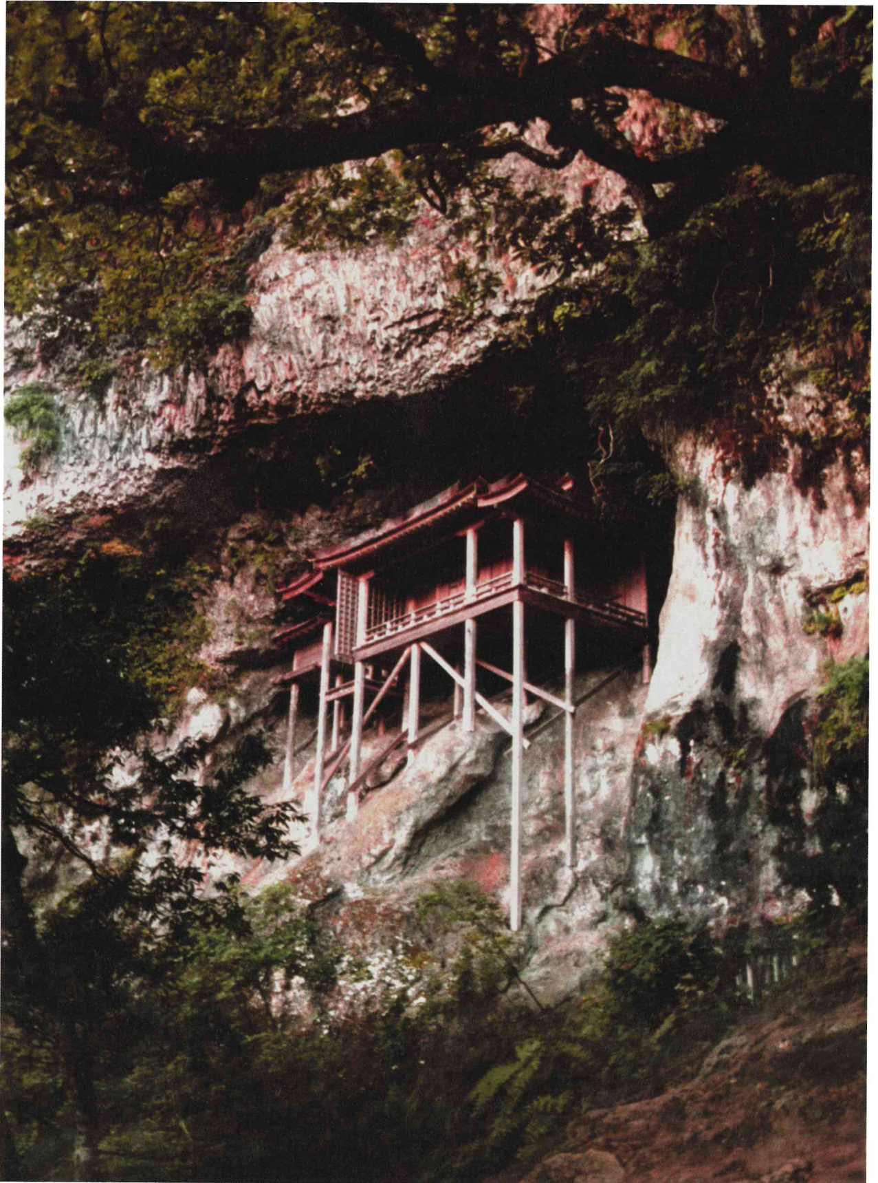
18 Built space honouring the spirit of a natural place. The Nageire-dou, Temple of Sanbutsu-ji, Tottori
