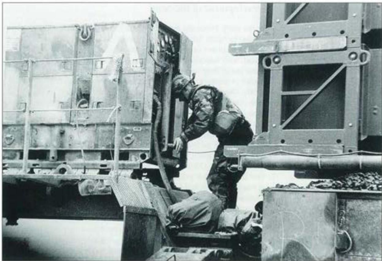
Starting one of two Patriot generators
