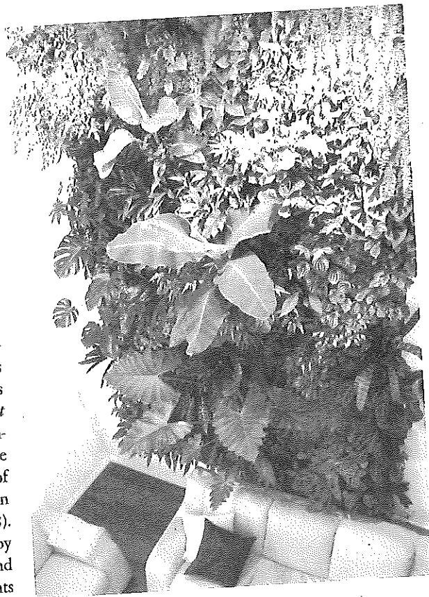
Fig. 4.1: Living walls or green walls are vertical gardens attached to the exterior or interior of a building. They do more than just beautify — they actually help improve air quality. This "Apartment therapy" by Green over Grey in a West End Vancouver loft incorporated 892 plants from 85 species into an 8'-by-16' wall. (CREDIT: MIKE WEINMASTER, GREEN OVER GREY, LIVING WALLS AND DESIGN INC.)
