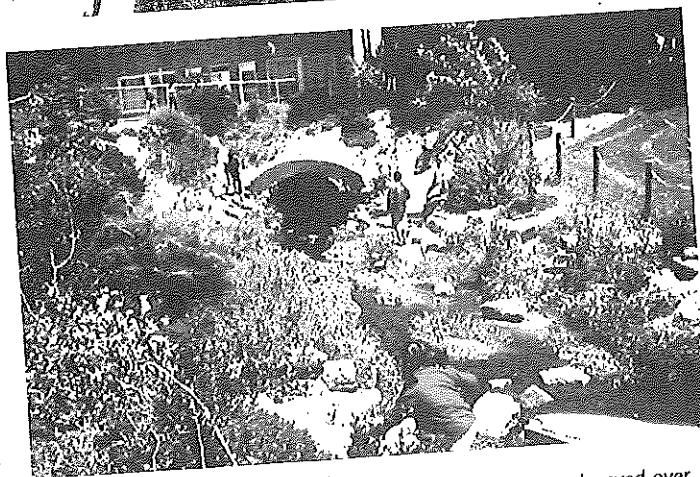
Fig. 4.4: Creek "daylighting" projects restoring formerly culverted, paved-over streams back to a more natural state to improve aesthetics, increase wildlife habitat, improve water quality and help stormwater surges in urban areas.
