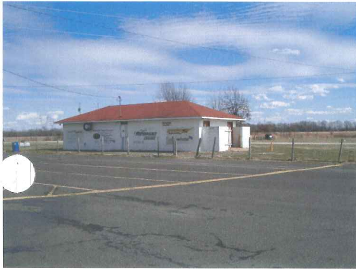
staging area & concession and restrooms
