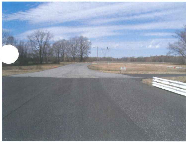
Light pole to be protected at shutdown return road side
