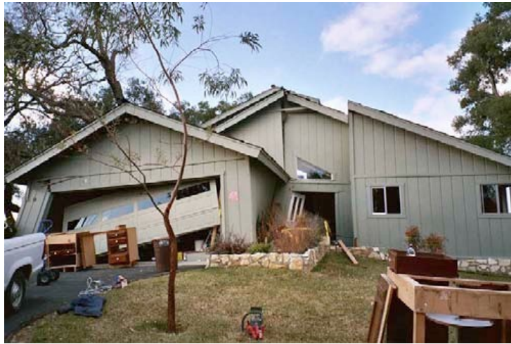
FIGURE 2-2 Atascadero, California, January 25, 2004. This home slid two feet off its foundation due to the 6.5 San Simeon earthquake.
