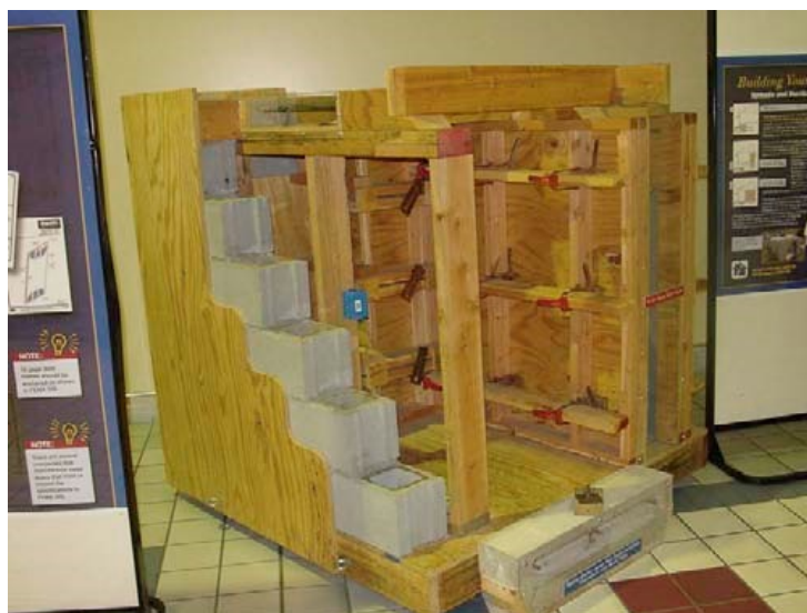
FIGURE 2-4 Tulsa, Oklahoma, November 23, 2001. Disaster Ally in the Eastland Mall. Safe rooms can be designed with many different materials. Shown are concrete block walls, formed concrete walls, and a special ceiling framing. Photo by Kent Baxter/FEMA News Photo.
