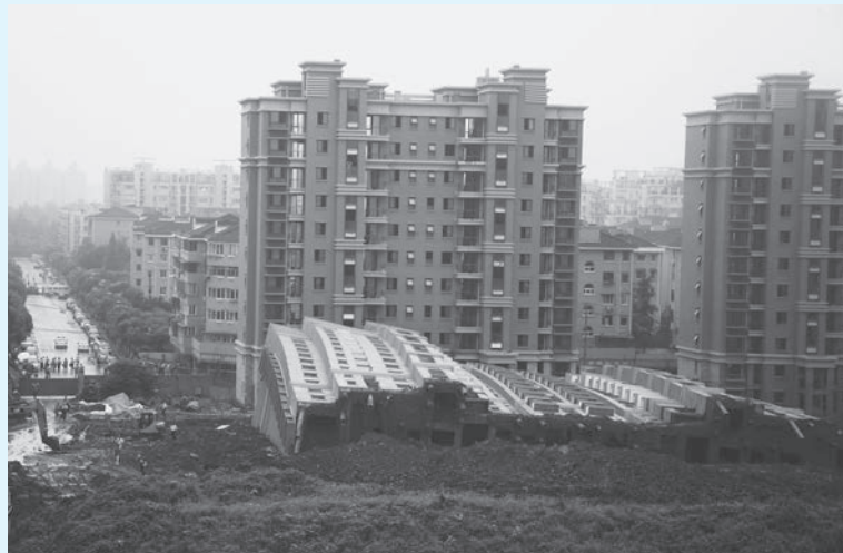
FIGURE 7.8 Shanghai Apartment Building Collapse
