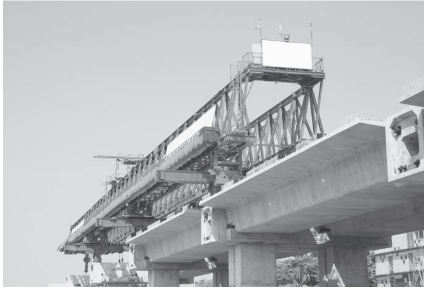
FIGURE 13.18 Honolulu's Elevated Rail project
