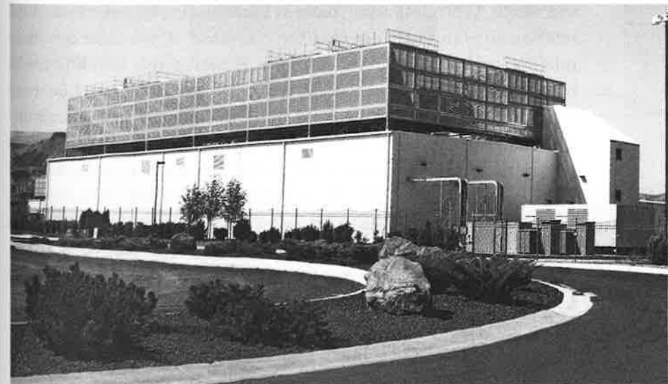
Google's data center complex outside The Dalles, Oregon. Photograph by the author.
