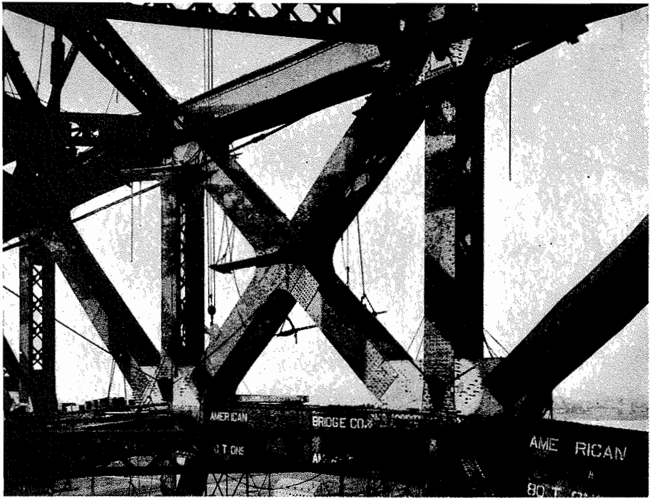
STEEL CONSTRUCTION. THE STEEL CORPORATION
