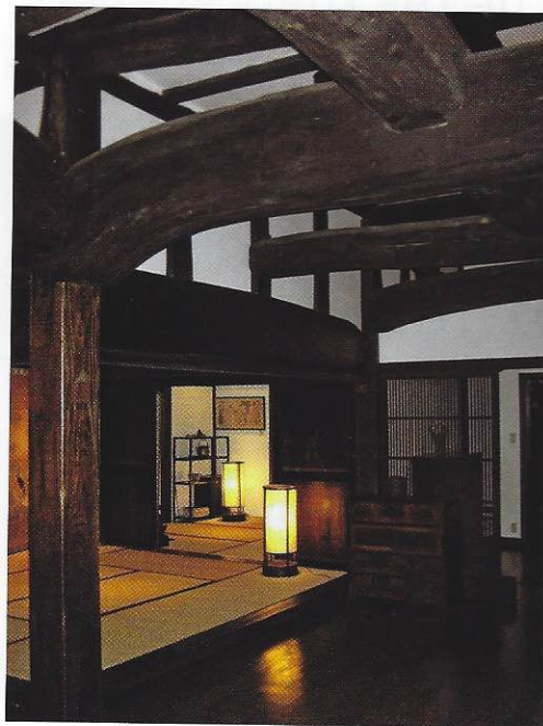
Plate 1-56 (right) Interior view of the Takishita House, Kamakura , renovation dating to 1976; originally constructed early 19 th century; moved and restored by architect Takishita Yoshihiro (b. 1945). Takishita has made a career of saving old minka (farmhouses) from demolition by moving those that cannot be preserved in situ and using their skeletal framework to create comfortable modern houses for himself and clients worldwide. Originally a village chief's house from a town in Fukui Prefecture, this large minka features posts made of keyaki (Japanese zelkova) and massive curved beams from giant old pine trees.
