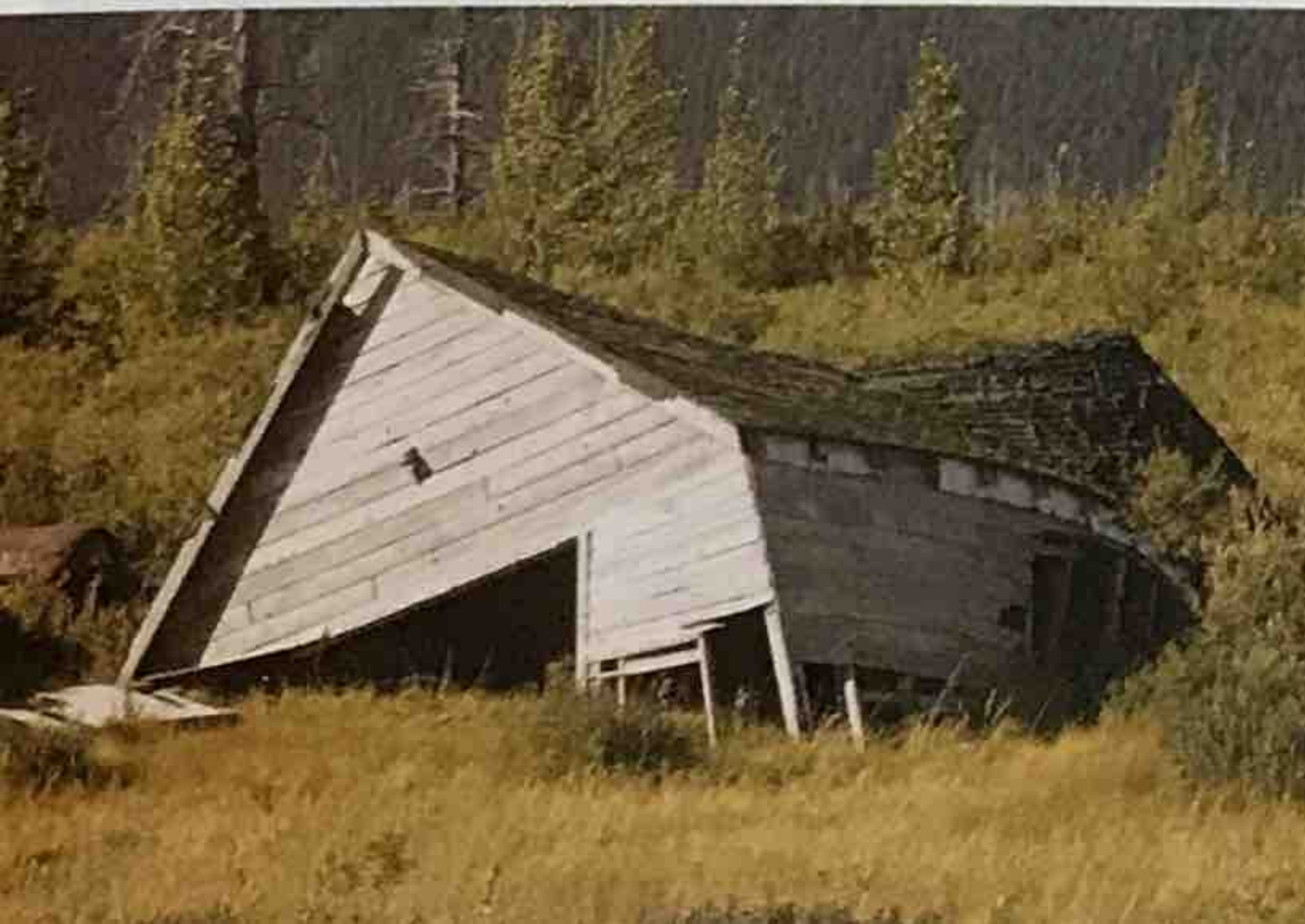
▼ Figure 9-18 House in Alaska collapsed as a result of melting permafrost.
