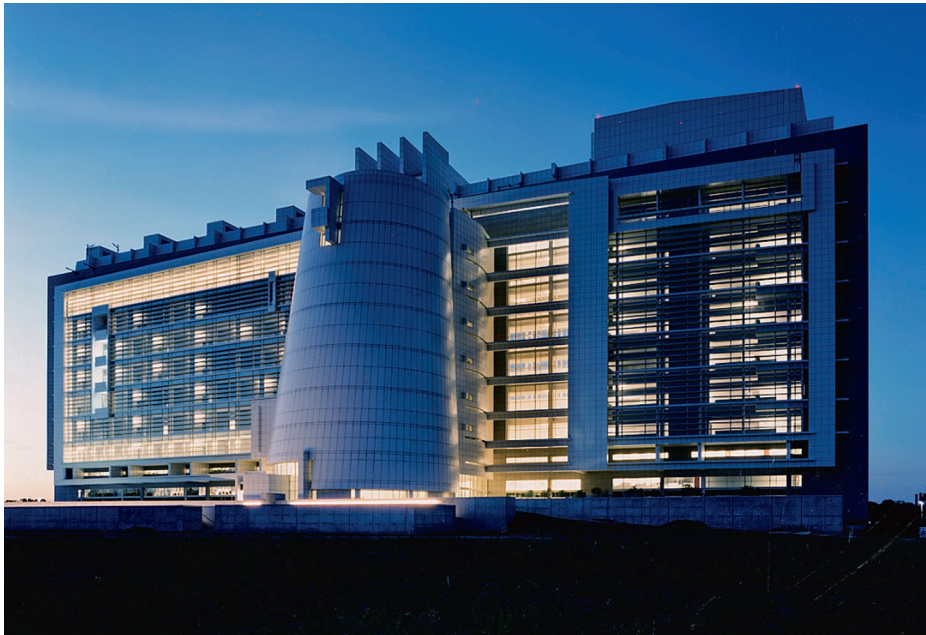
FIGURE 6-23 Richard Meier, Long Island Federal Courthouse, Central Islip, New York. 2000. A stark white building, it is one of the largest courthouses in the nation. It is designed to accommodate public gatherings as well as numerous individual courts.
