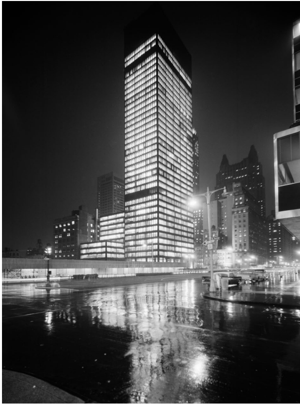
FIGURE 6-6 Ludwig Mies van der Rohe and Philip Johnson, architects, the Seagram Building, New York City. 1954–1958. An example of the International style popular in midcentury, the building was designed so that the structure of the building would be visible. Without decoration, and with replication of floor upon floor, this building reveals a clear function for “doing business.”
