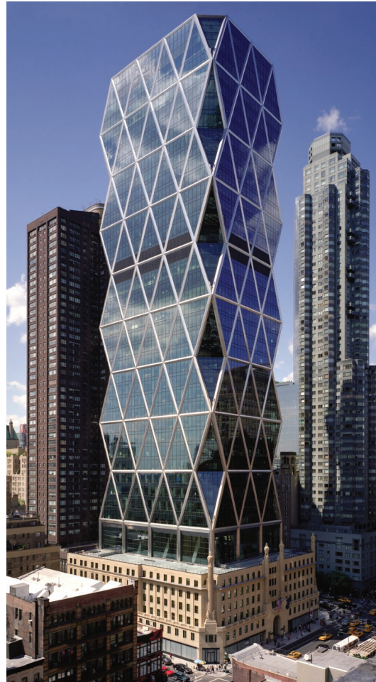
FIGURE 6-32 Norman Foster, Hearst Tower, New York City. 2006. The project was to build on top of a seventy-eight-year-old limestone building whose interior was essentially gutted to accommodate the tower, which rises sharply and suddenly above the conventional lower section.
