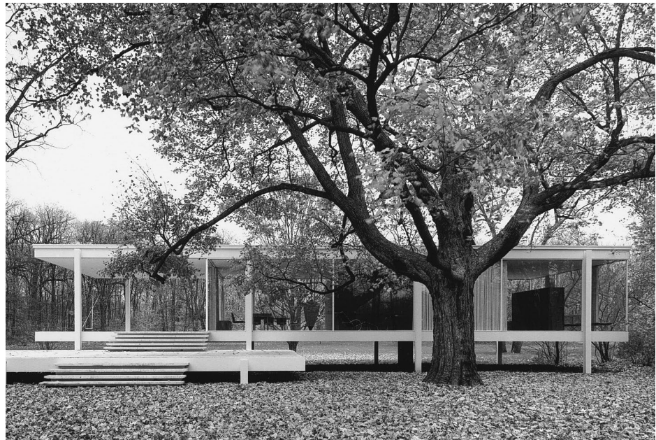
FIGURE 6-20 Ludwig Mies van der Rohe, Farnsworth Residence, Plano, Illinois. 1950. Mies insisted on building with the interior structure visible from all angles.
