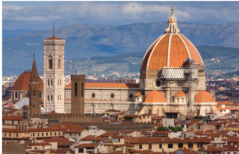
FIGURE 6-18 Filippo Brunelleschi, dome of the Cathedral of Florence. 1420–1436. One of the great architectural achievements of the Renaissance, the cathedral still dominates the landscape of modern Florence.
