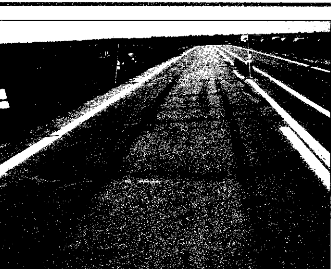
FIGURE 11. Improper photographic technique: Vehicle ending point is not visible
