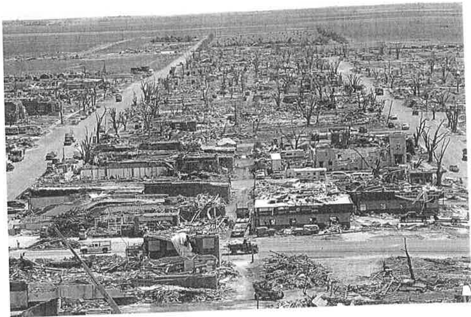
Figure 16-5 The center of Greensburg, Kansas, twelve days after being hit by an F5 tornado with 200-mph winds on May 4, 2007
