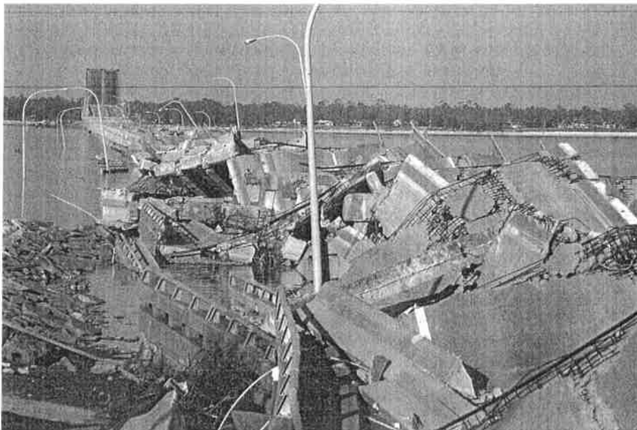
Figure 16-2 Highway 90 bridge from Biloxi to Ocean Springs, Mississippi, after Katrina's catastrophic winds and storm surge
