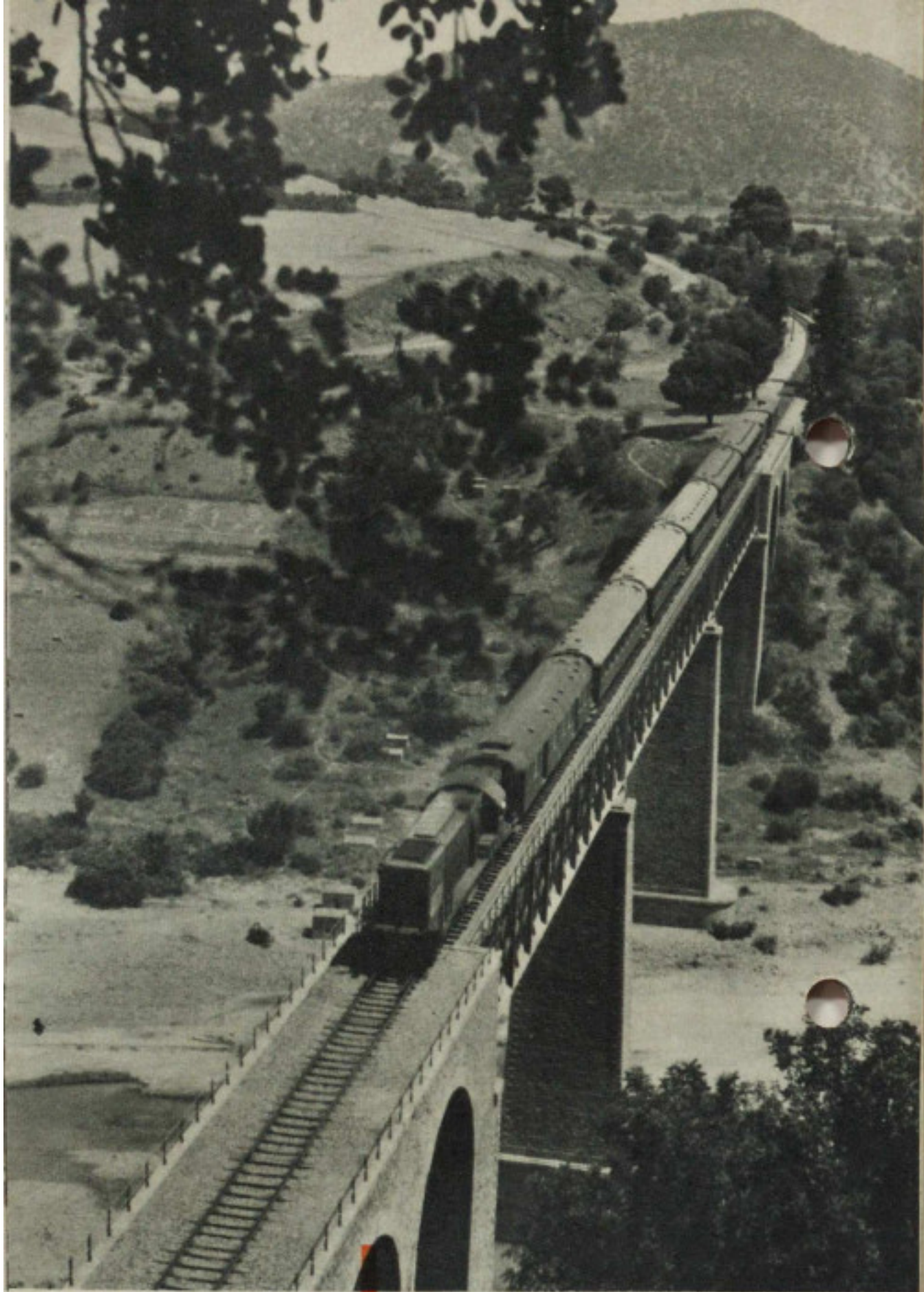
The railway bridge and road in the gorges of Beni Amran.
