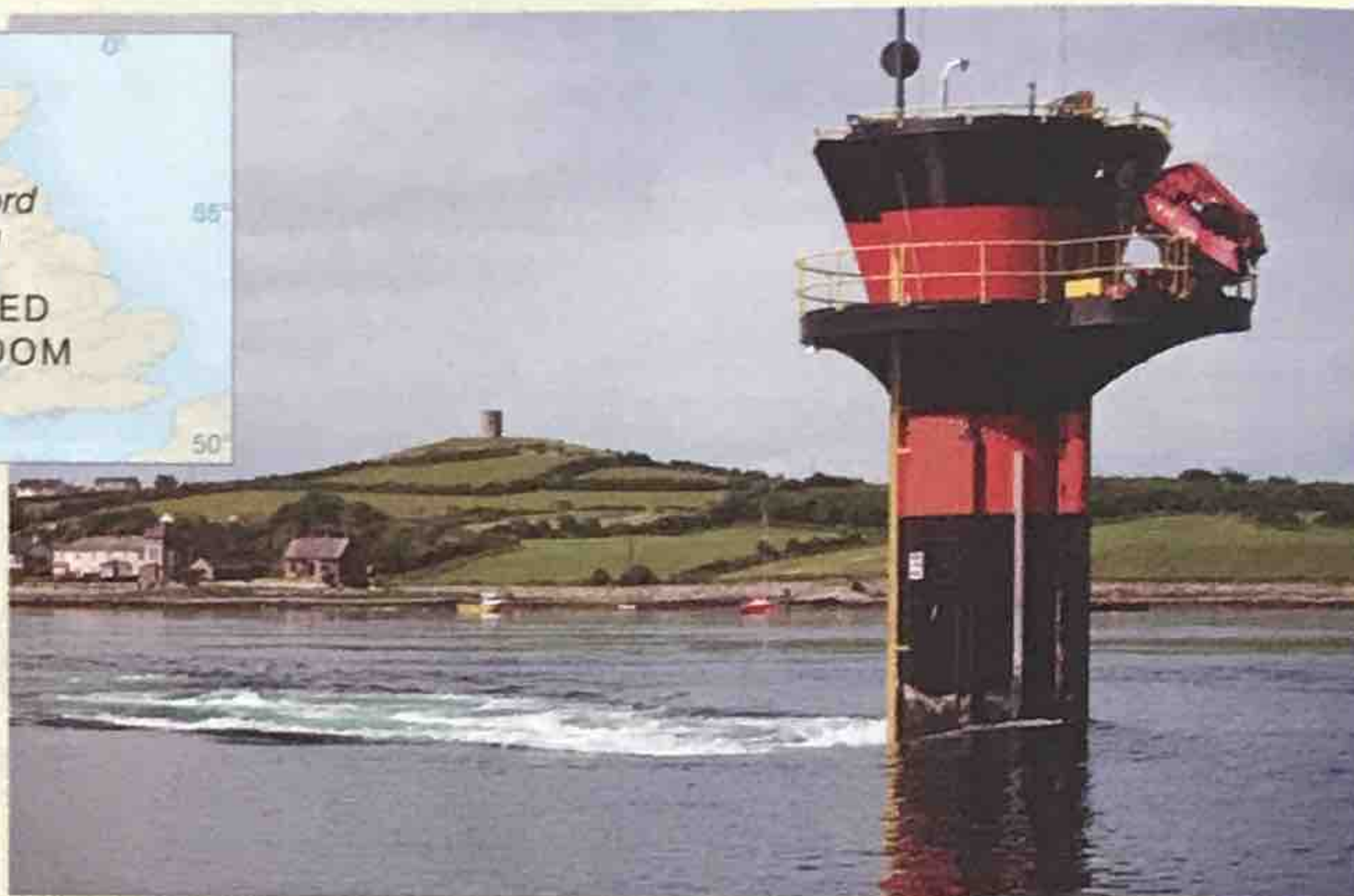
▲ Figure 20-E Tidal power turbine in Strangford Lough, Northern Ireland.
