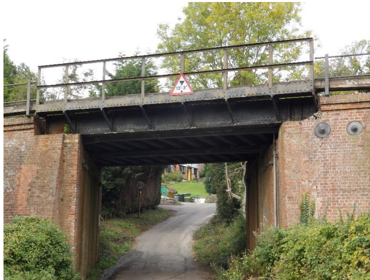
Figure Q1(a)A Plate Girder Bridge in Need of Replacement
