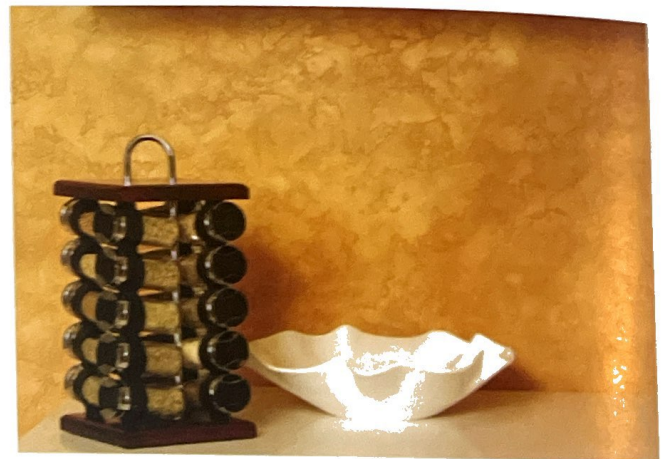
Figure 3.10 Tactile textures, such as those found in nature, may be enhanced by age or simulated with faux painted techniques, such as Venetian plaster. ( Decorfin )
