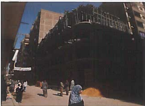
In Egypt, builders often leave the top floor of new construction unfinished to avoid paying property taxes.
