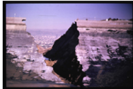
Figure 2-1. San Fernando Valley, California, viewed through a breach in the Van Norman Dam after the 1971 earthquake. (Courtesy of the Los Angeles County Fire Department, Los Angeles, California.)
