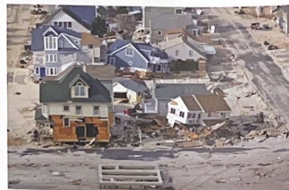
Destruction by Hurricane Sandy on Ortleigh Beach, New Jersey. Hurricane Sandy, moving ashore in New Jersey on October 29, 2012, was the second-costliest hurricane in U.S. history. Its high winds struck twenty-four states, including the entire eastern seaboard from Florida to Maine.
