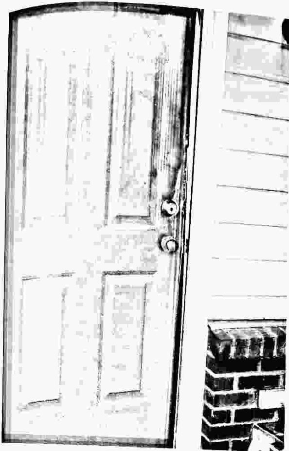
◀ FIGURE 14-3 Broken front door
