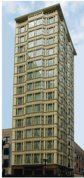
▲ 26-5. Reliance Building, 1890–1894; Chicago, Illinois; Daniel H. Burnham and John W. Root.
