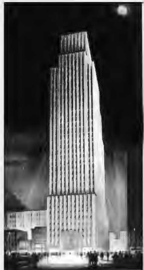
Figure 2.45 | New York Daily News Building
