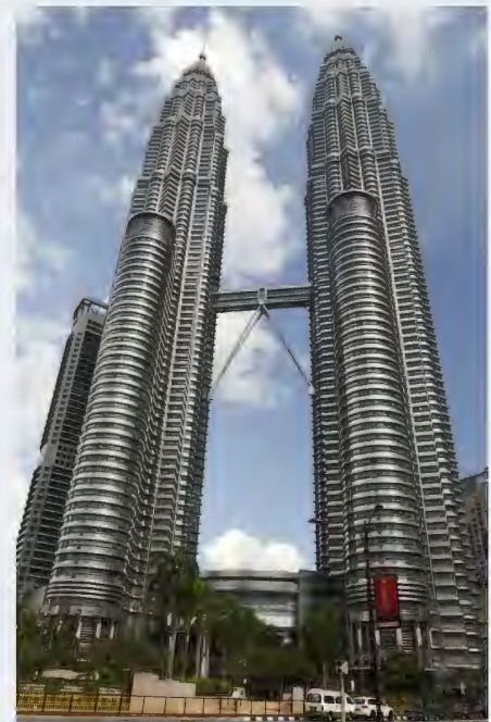
Figure 7.38 | Petronas Twin Towers, Malaysia
