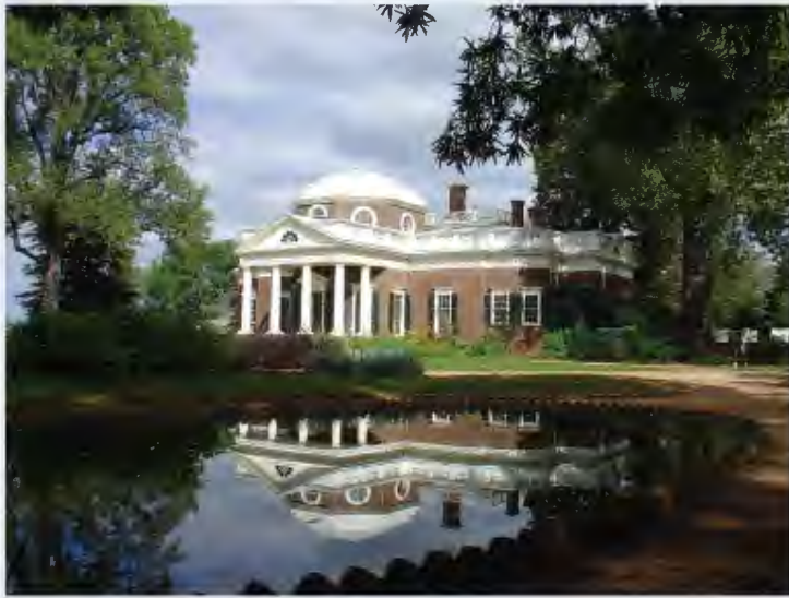
Figure 7.19 | Monticello, Charlottesville, VA
