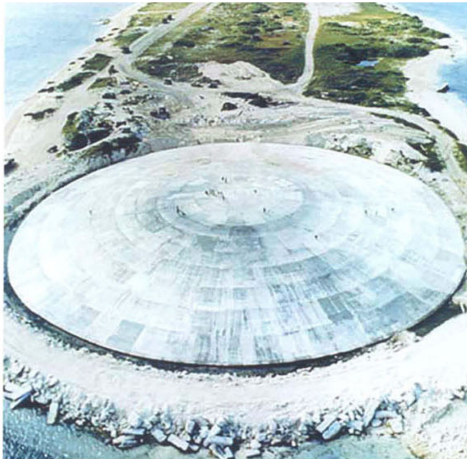
The Runit Dome on Enewetak was constructed in the late 1970s. The United States bulldozed some 11,000 cubic yards of radioactive topsoil and debris into a crater from a nuclear bomb test and then sealed it over with concrete in an attempt to contain radioactivity. Is seawater leaching underneath the Runit Dome and transporting radioactive compounds into the ocean?
