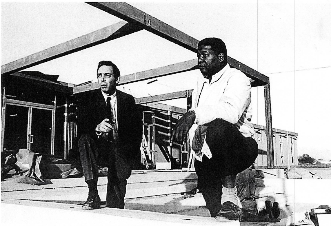
H. Jack Geiger (left) and John Hatch (right) during the construction of the Tufts-Delta Health Center, Bolivar County, Mississippi, in 1966. Photo courtesy of Dan Bernstein. Printed with permission.
