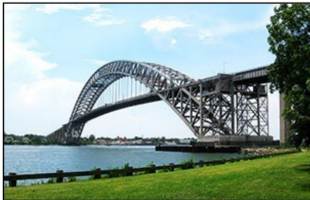
FIGURE 2 Built in 1931 to accommodate a 151-foot clearance over the Kill Van Kull waterway between New Jersey and New York, the roadbed of the Bayonne Bridge was raised in 2019, under a joint venture, to 215 feet, to handle post-Panamax ships. [Photo credit: Bayonenju.org]
