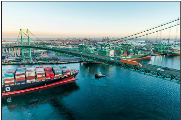
FIGURE 23 Approximately forty percent of all containerized cargo in the U.S. and nearly half of all the oil imports for the U.S. west of the Rocky Mountains arrive via the Ports of Los Angeles (above) and Long Beach. Due to the “just in time” philosophy of modern shipping, there is often just two weeks of refined fuel available to serve the entire Southern California economy. Thus, a disaster that impacts the functioning of these ports, even for a relatively short time, would have catastrophic impacts on millions of people. Photo Credit: Port of LA
