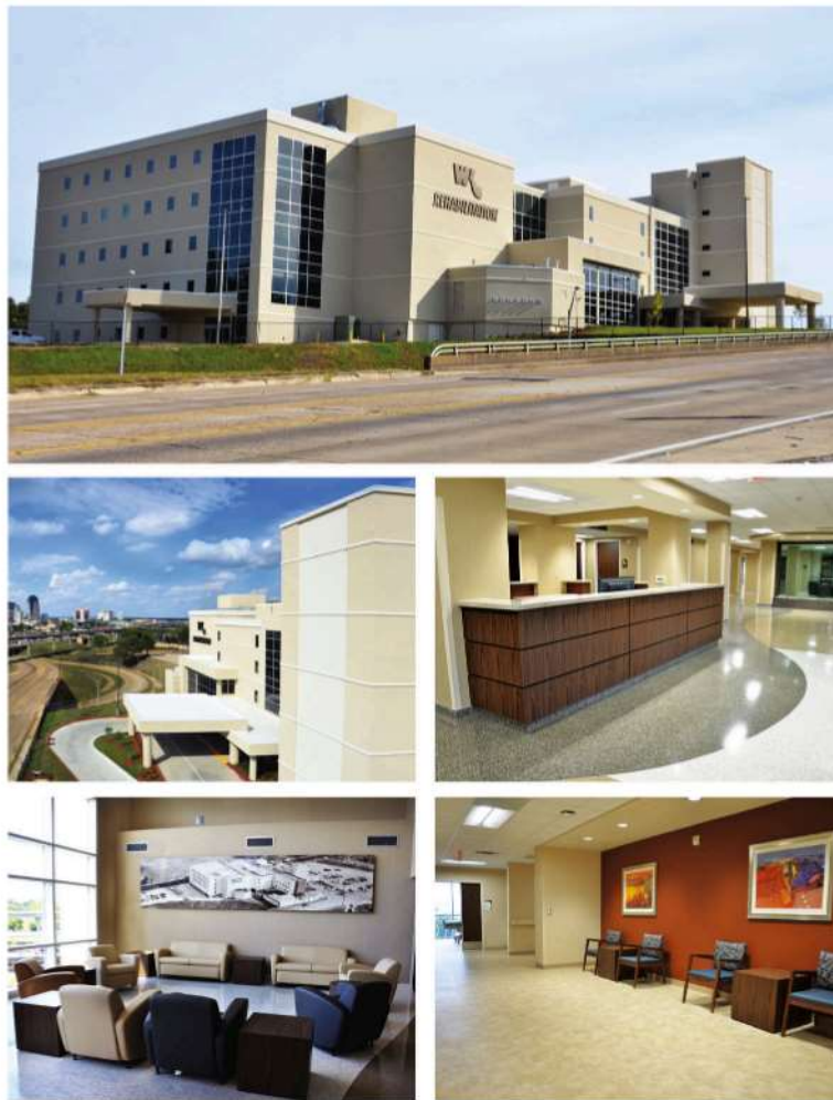
Fig. 2 The WK Rehabilitation Institute, repurposed from Doctors' Hospital. Copyright © 2016 Willis-Knighton Health System. Used with permission. The dramatic adaptive reuse transformation of the former Doctors' Hospital of Shreveport into Willis-Knighton Health System's newest center of excellence, the WK Rehabilitation Institute, is clearly presented in the noted photographs. The resulting building, reintroduced in 2017, is virtually indistinguishable from brand new construction and features an entirely revised facade, all-new interior elements, and an enhanced layout which facilitates access. A property that once blighted the community now serves as a symbol of innovation and progress
