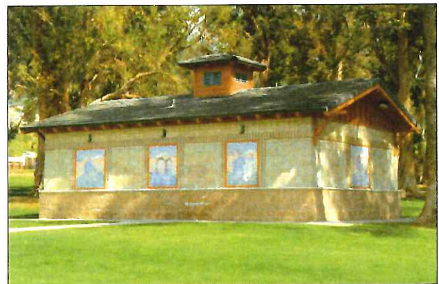
Pioneer Park Restroom Building
