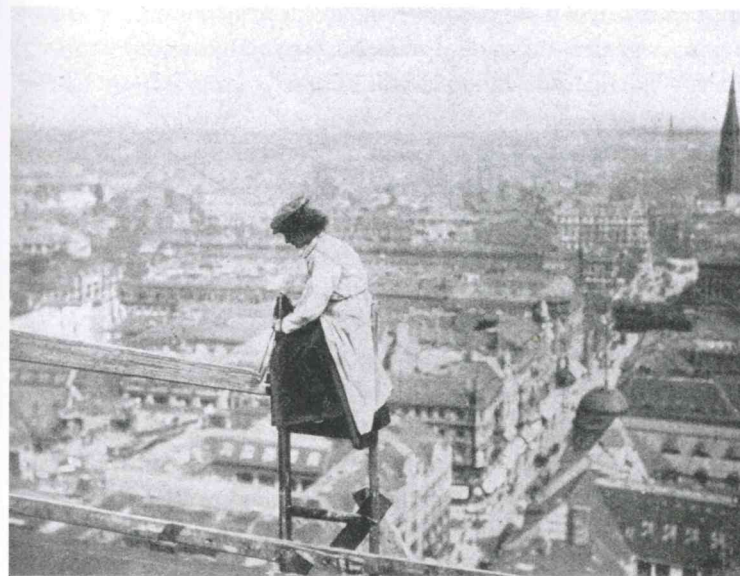
2. Recalling Fay Kellog in New York City, a woman builder in Berlin shows off her daring for the press. She is pictured making repairs to the roof of Berlin's City Hall in 1910.
