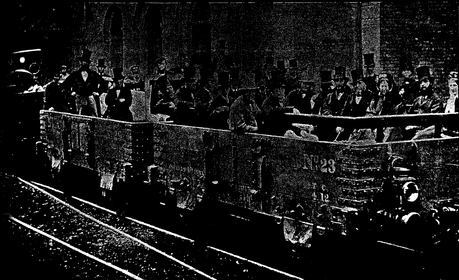
The first underground steam train: the inaugural trip on the first section of the Metropolitan Line from Edgware Road on 24 May 1862, before it was opened in 1863; the passengers included Gladstone and his wife.
