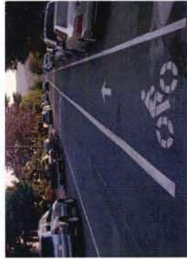
FIGURE 8 Bike lane striping and stencil
