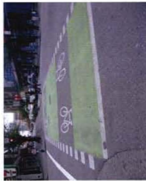
FIGURE 2 Cycle track intersection treatment.
